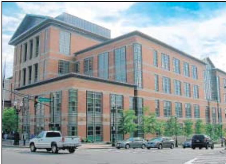
Cleanup of the site on which the new Worcester Trial Court now sits is one of the latest feathers in the cap of OTO; the firm focuses not only on large, high-profile commercial, industrial and governmental projects but smaller jobs too.
